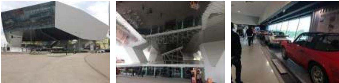
Figure (24) Porsche Museum curtain wall & podium
